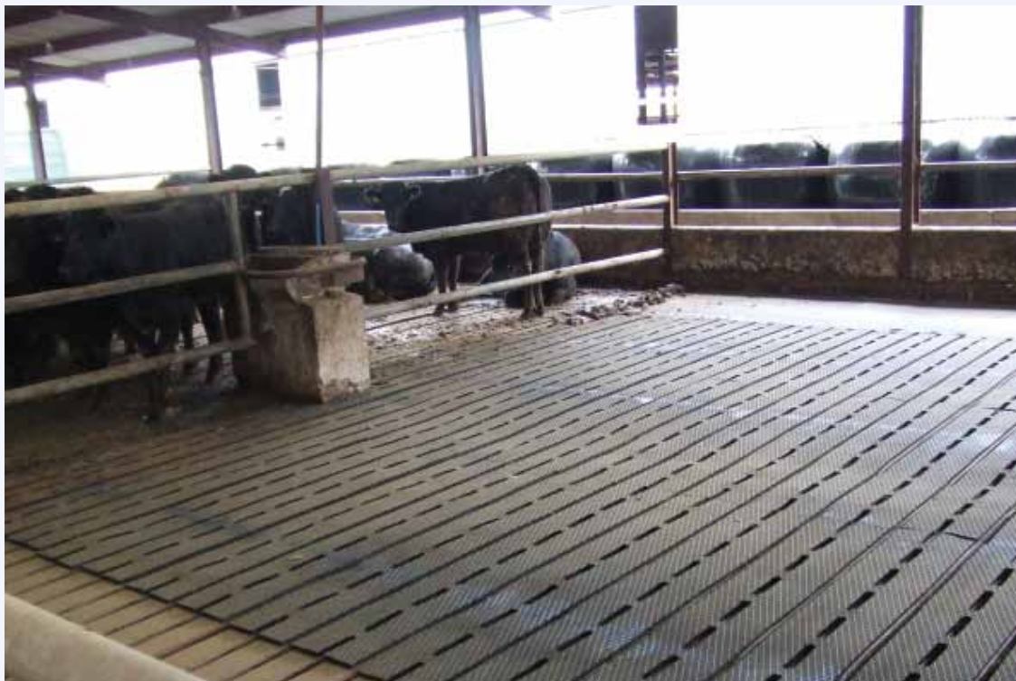
RUBBERISED SLATS OVERLAY CONCRETE SLATS ARE EASY WITH QUICK BENEFITS FOR WELFARE
