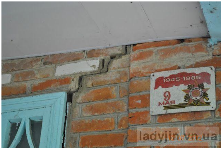
Cracks have appeared in almost every house in Olyanytsva's main street since MHP began expansion of its Vinnitsa complex. Residents blame heavy lorry traffic.
